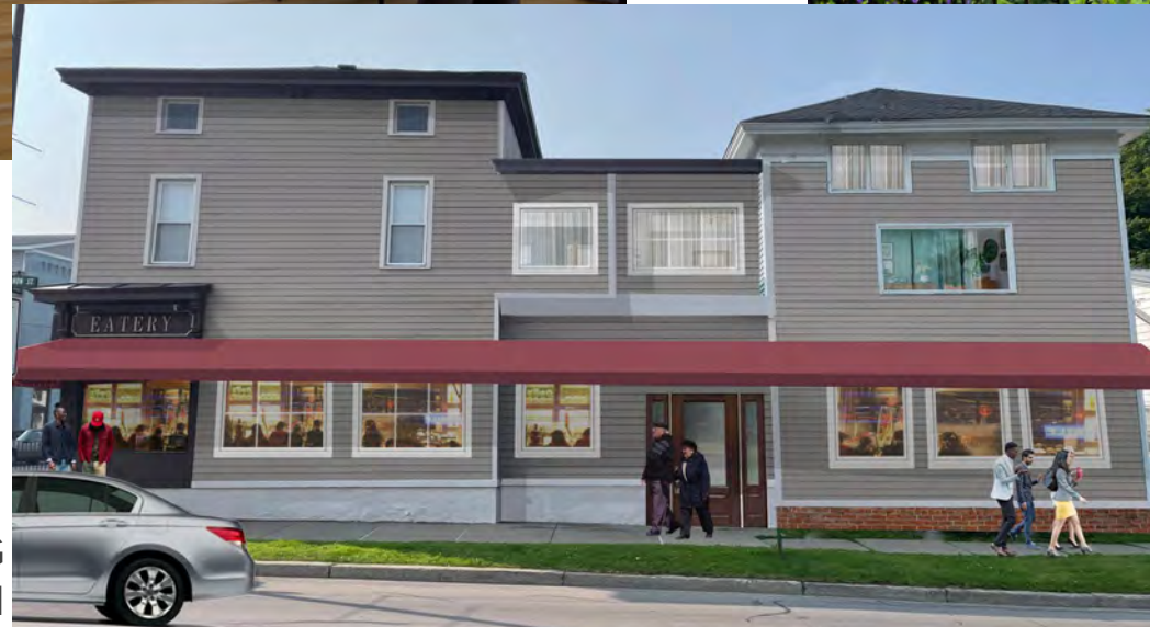
MIXED-USE BUILDING RENOVATION
